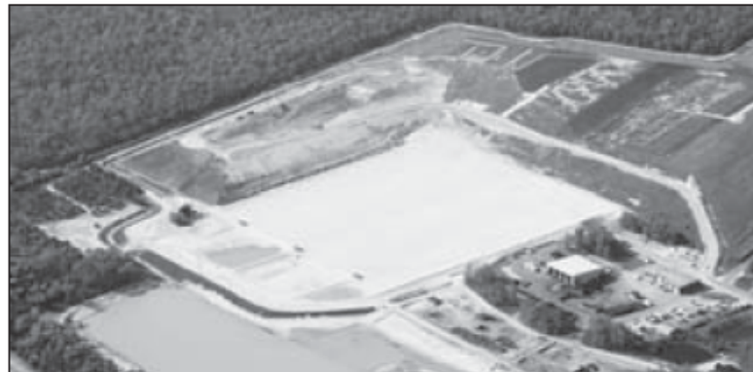
Aerial view of new Cell F ready to be filled at county MUA's sanitary landfill. To the above left is Cell E and the capped fields are above to the right.
