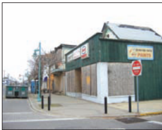
Burned-out buildings front Landis Avenue.
